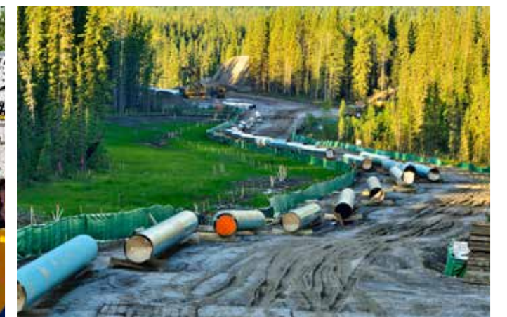
Laying out the Trans Mountain oil pipeline near Hinton Alberta Canada PHOTO: Robert McGouey / Industry / Alamy Stock Photo
